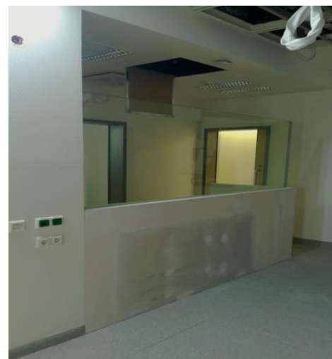
Radiation-shielding screen, as plasterboard model, with 90° angle:
