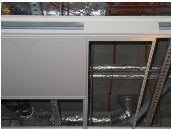
Heavy-duty ceiling with clip-in assembly, including installation frame for luminaire
