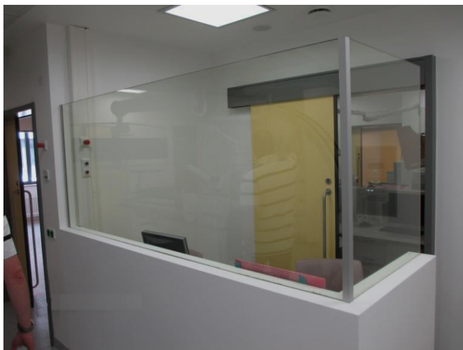
Radiation-shielding screen, as plasterboard model, with 90° angle:
