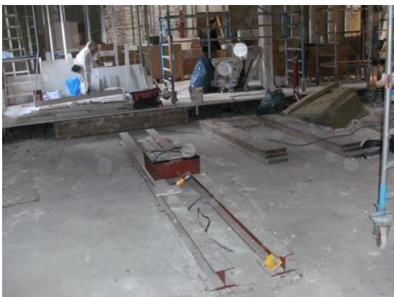
Floor plate on load-spreading supporting structure
