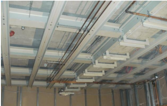
Installation of load-spreading steel assemblies
