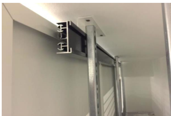
With variable suspension systems, all metal tiles at all positions are subsequently removable.
